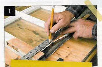
▲ 1. Start by assembling your tools: a straight edge, combination square, router and straight bit, ruler, wood chisel, block plane, epoxy, random orbit sander, and enough wood to create the patch. Ideally, the wood should be the same type as the original, and match its grain as closely as possible. Begin by laying out the area to be removed and marking the boundaries with a sharp pencil or utility knife.
