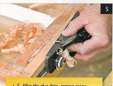
▲ 5. After the glue dries, remove excess material with a block plane and sand the patch smooth using a random orbit sander and 100-grit paper. Fill any cracks between the old and new surface with a filler, allow it to dry, and sand smooth. The repair is now ready for priming and painting.
