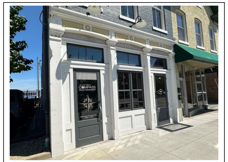
The design of the new storefront above utilizes large display windows with transom window, above a low bulkhead. Below, a new storefront was designed to fit within the historic limestone columns and cornice.
