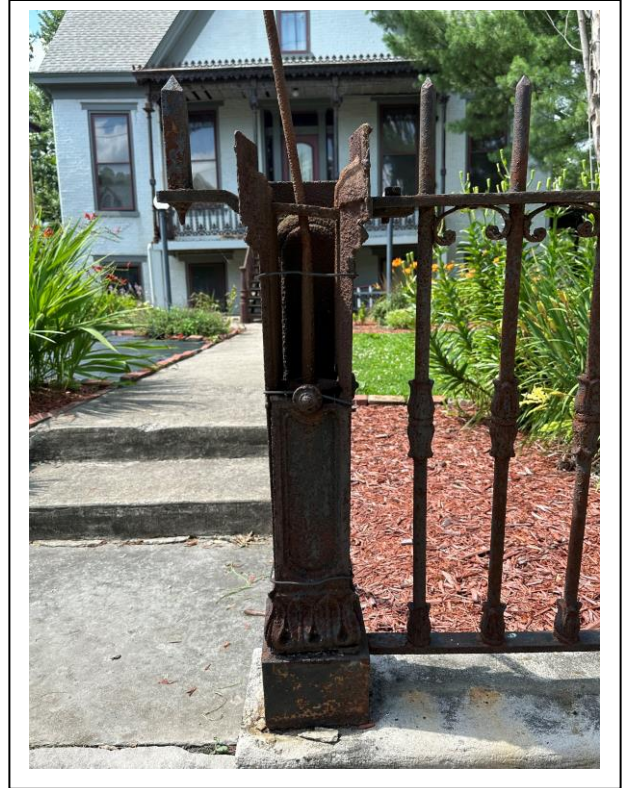
Cast iron is susceptible to water damage, which can lead to rust and cracking.
