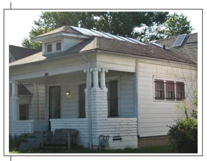
The solar panels in the above example would have been more appropriately installed in a less conspicuous location set back from the front plane of the house. The tangle of wires leading down from the panels is also not consistent with these design guidelines.
