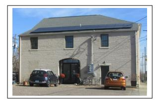
**AE7** For solar panels – if placed on the sloped roof of a structure, the angle of the solar panels should match the roof angle, and the panels should not extend beyond the edge of the roof on which the panels are installed. On flat-roofed structures, the panels should be set back from the roof edge to minimize visibility. Pitch and elevation should also be adjusted to reduce visibility from the public right-of-way. Total roof area covered by a solar installation should not exceed 90%.
