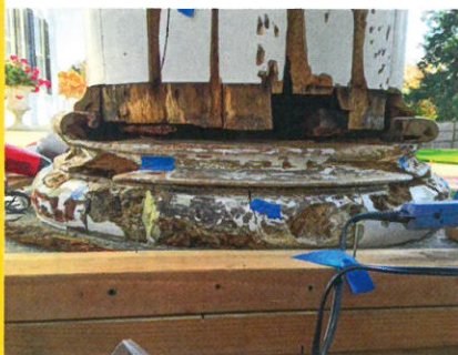
Repair of exterior columns using ConServ Epoxy products involved liquid borate preservative, epoxy consolidation, epoxy filling and shaping, and new wood at the base.
