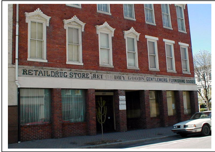
Historically, signs were often located in the storefront cornice area, as seen on this Pearl Street building.
