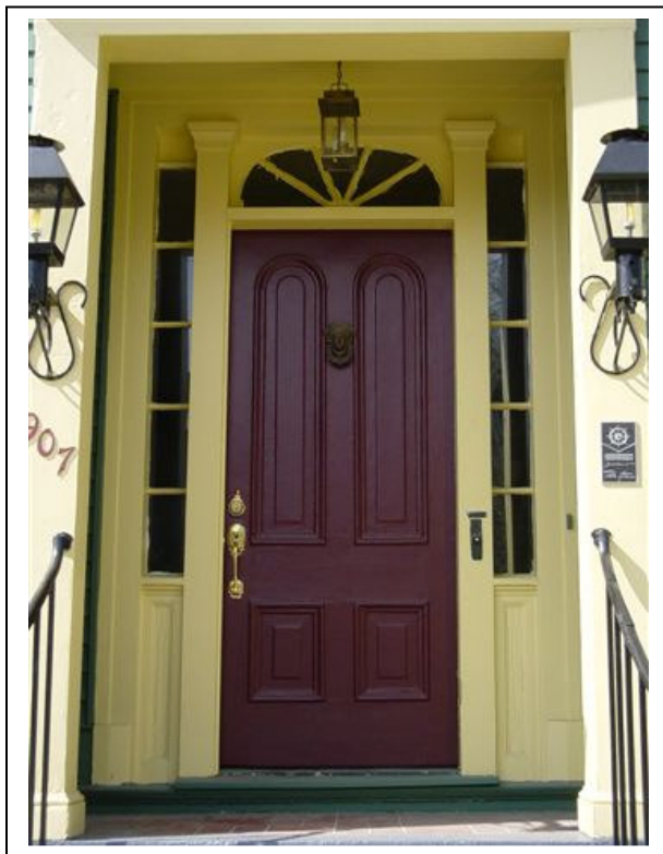
The fanlight and sidelights around this door on East Main Street is an important part of the building's historic character.
