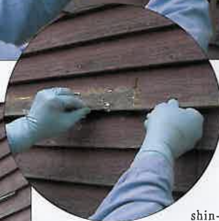
Left: Remove the patch, apply waterproof glue to all edges, then clamp in place with slim wedges.
