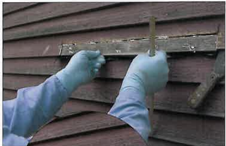
Left: Remove the patch, apply waterproof glue to all edges, then clamp in place with slim wedges.
