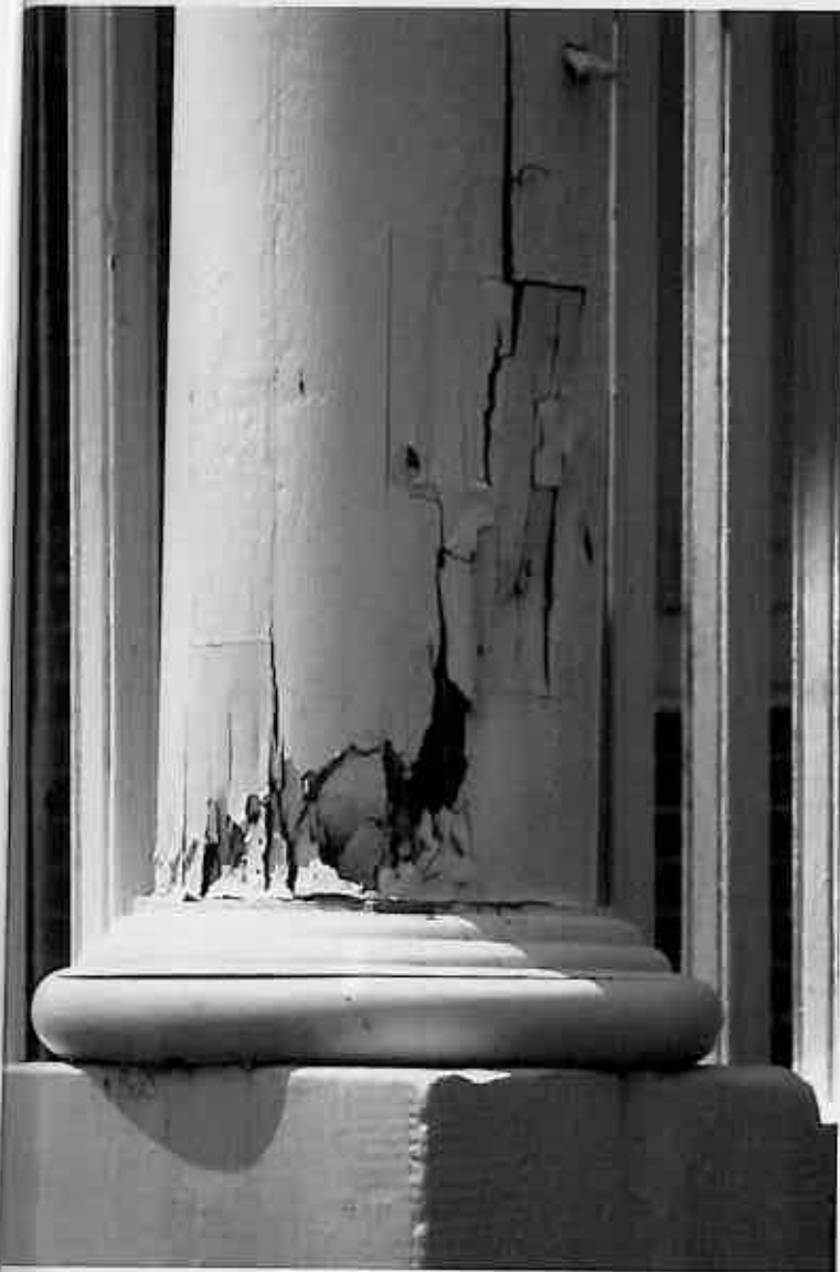
LEFT: Water seeping into hollow, unvented columns can create a breeding ground for mold; simple vents at the top and bottom of the column will allow water to evaporate.
