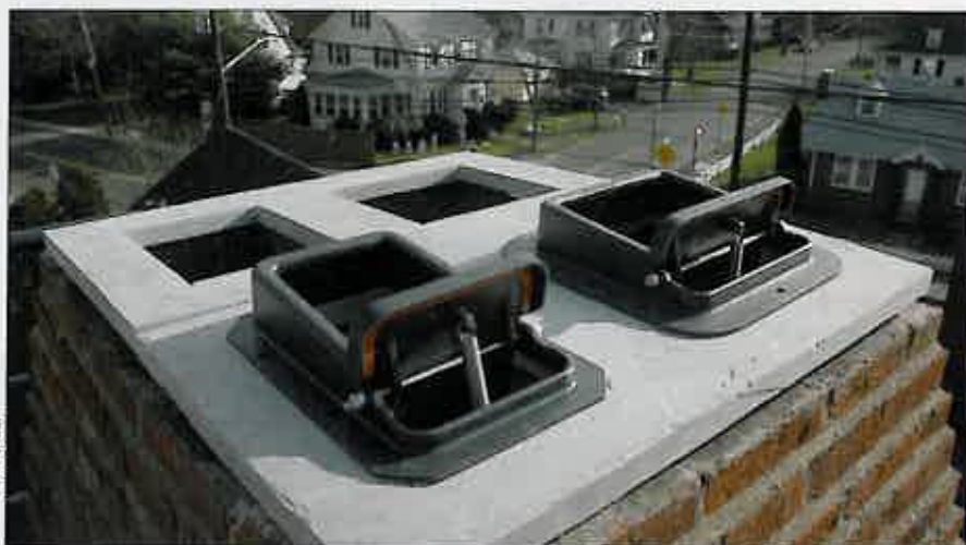
Adding exterior, top-mounting dampers (above) to these 180-year-old fireplaces sealed them with minimal disruption. Daylight shining through a rubble foundation (right) is a sure sign of an air leak that needs attention.
