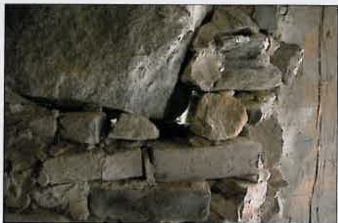
Adding exterior, top-mounting dampers (above) to these 180-year-old fireplaces sealed them with minimal disruption. Daylight shining through a rubble foundation (right) is a sure sign of an air leak that needs attention.
